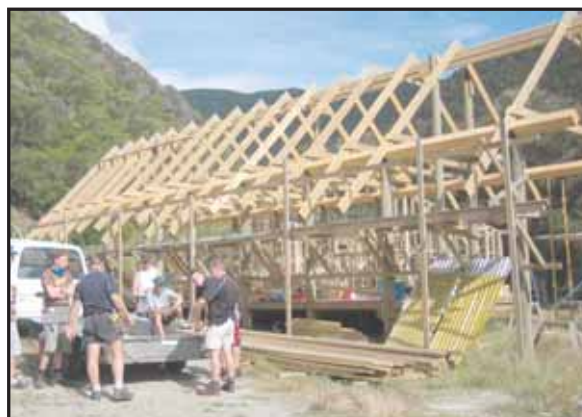
NMIT students & staff carry out roof preparation
