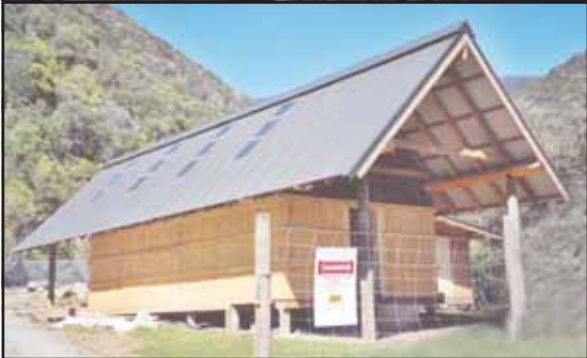
Interior & exterior of Entrance Building
